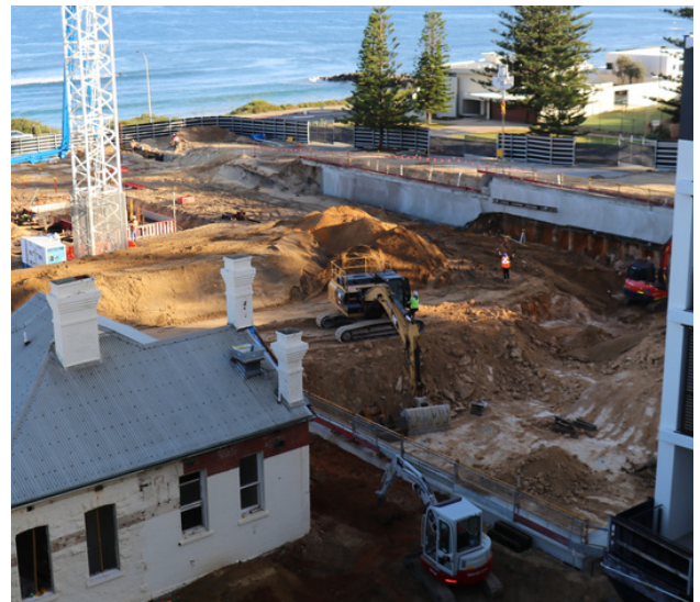
Bulk earthworks - looking north west
